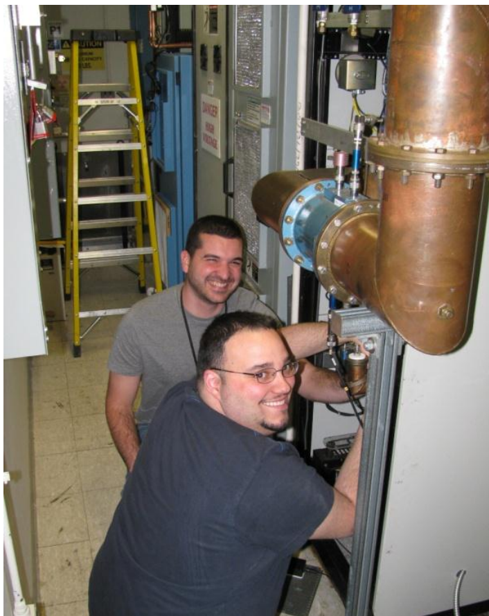
Completing the RF connections to the 123kW amp
