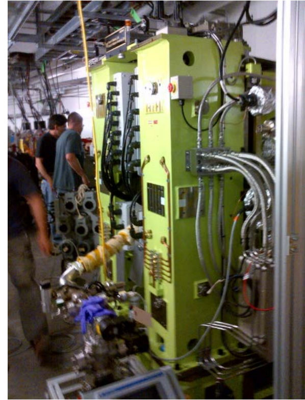
HXN IVU during installation
